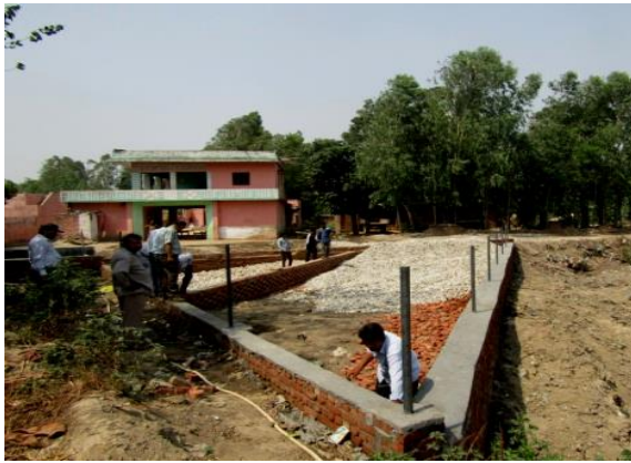
b: Establishment of CW in pond with connecting sedimentation chamber
