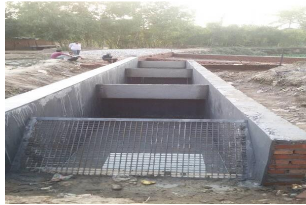
b: Establishment of CW in pond with connecting sedimentation chamber
